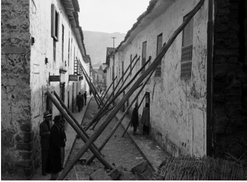
Figure 1. Cusco Earthquake damage, 1950. (Credits: LIFE historic file).
