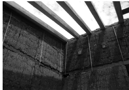
Figure 4. Connected collar beams (Centro Tierra).
