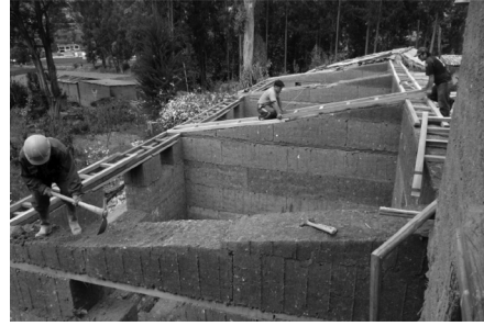
Figure 3. Introducing collar beams (Centro Tierra).
