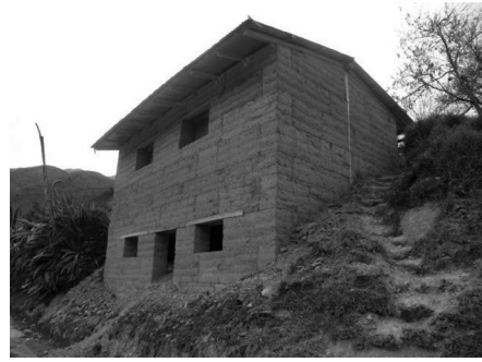
Figure 2. Traditional rammed earth house (Centro Tierra).
