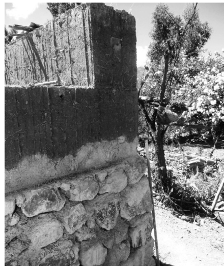
Figure 5. Reinforced foundations with lime mortar (Centro Tierra).
